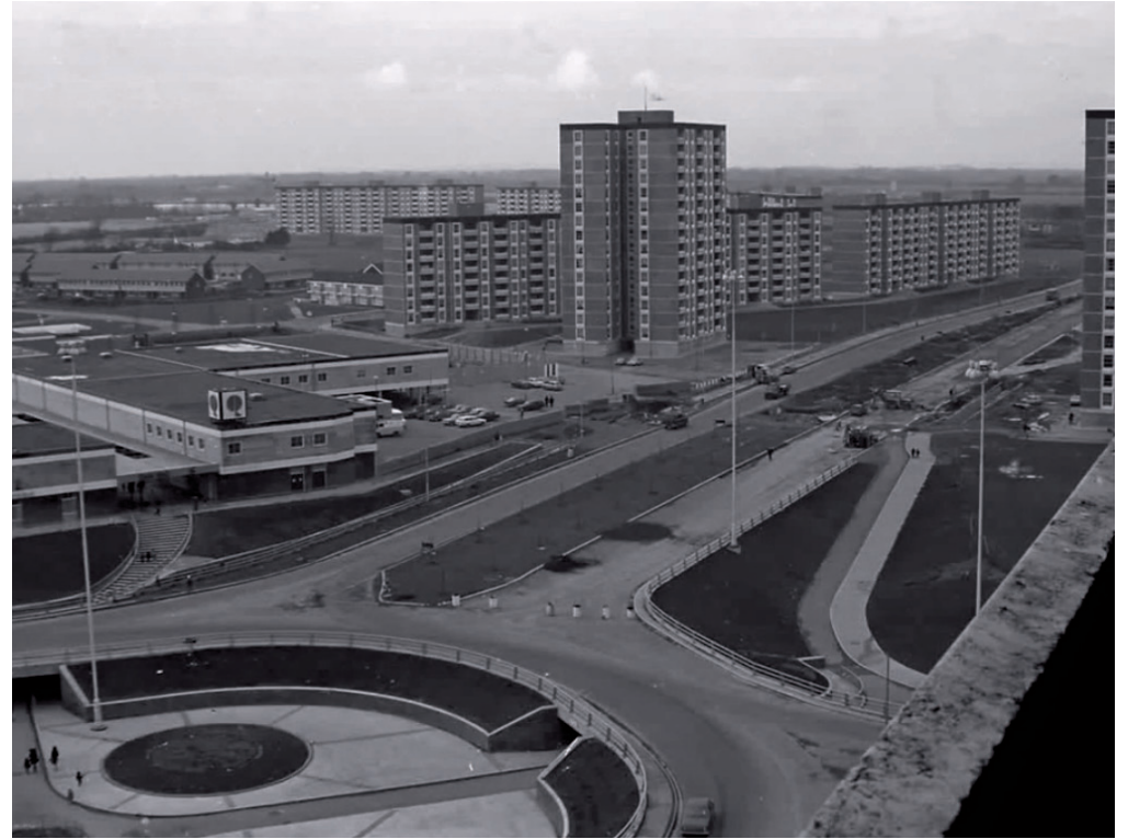
View to Ballymun tower block and main road.
