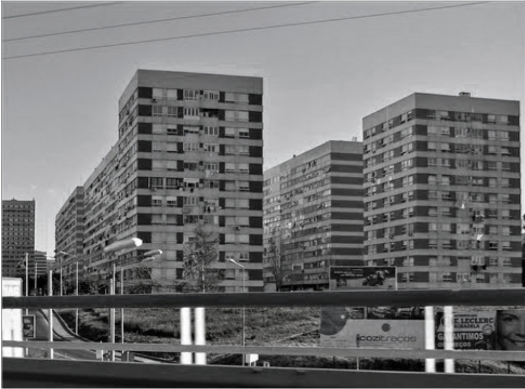
View to Portel housing scheme large slab blocks
